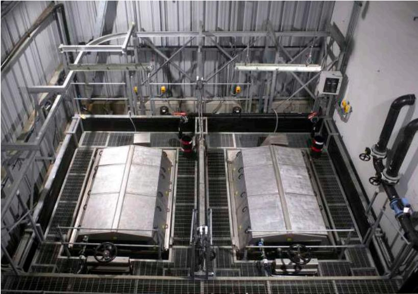
Another challenge that required some innovation was the need to install recirculation technologies in an existing, and limited, space in the fry room, which was formerly used as a feed warehouse. A very compact version of Billund Aquaculture's RAS systems had to be installed, while a fiber-reinforced plastic biofilter was used instead of a concrete one which would have taken longer to build in this very rainy location.
